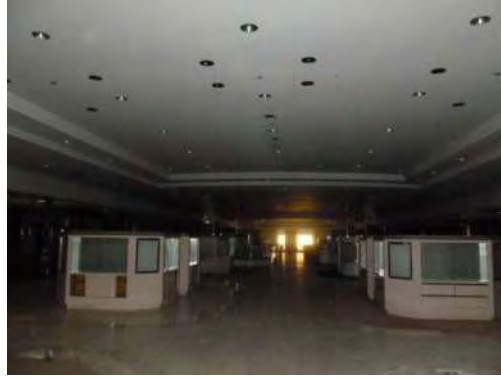
Macy's – carpet and tile with gypsum wall board ceiling
