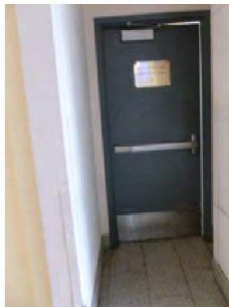
typical back of house hollow metal door
