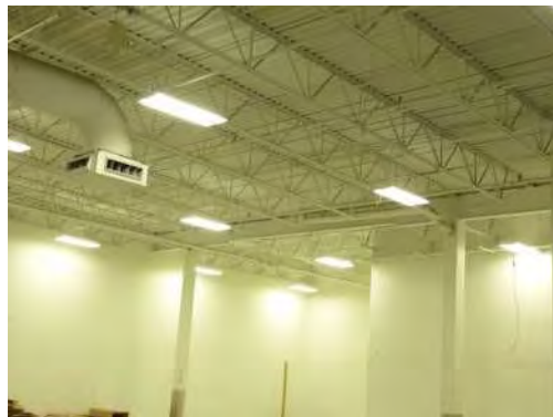
Best Buy roof structure
