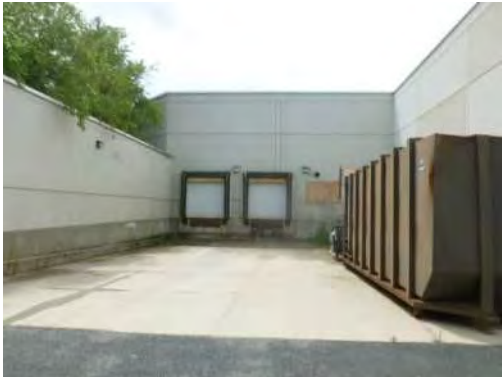
overhead doors at Macy's
