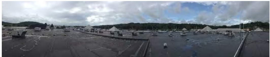
panoramic of the main roof
