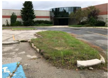
Site Photo Taken by MMI—Aug. 22, 2018
