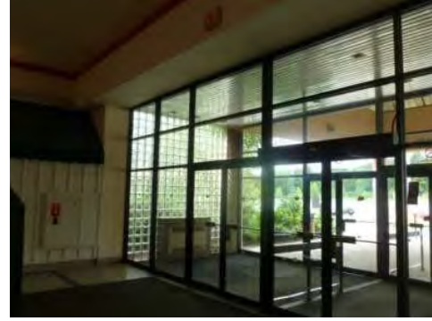
glass block at entrances
