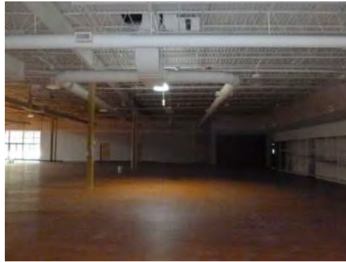
retail space, open to structure
