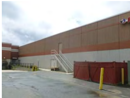
typical painted ribbed CMU
