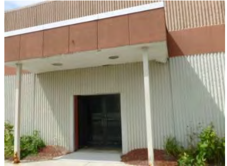
painted CMU and EIFS at Sears
