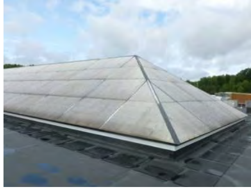
hipped panel skylight
