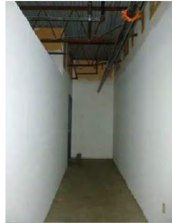
back of house second floor corridor
