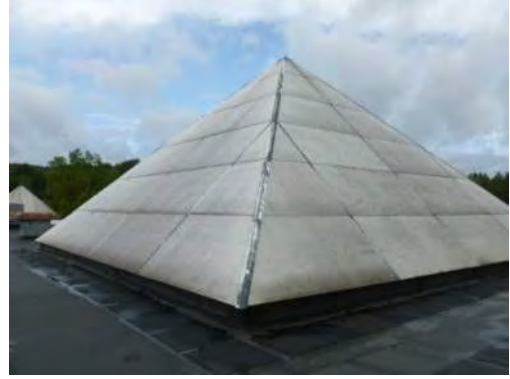
pyramid panel skylight
