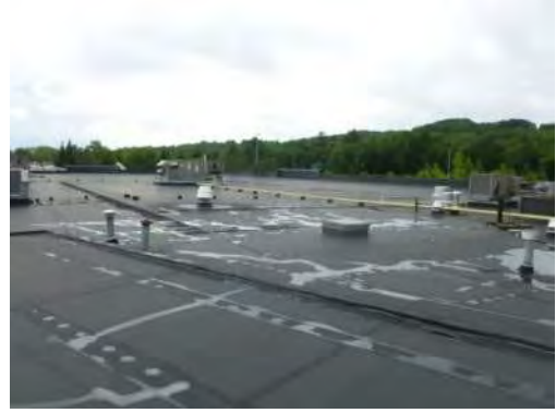
roof has both many penetrations and equipment on sleepers
