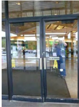
typical original entry doors
